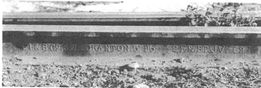
Out of the past! This bit of relay rail on an M. & E. T. siding is from the original San Francisco & San Joaquin Valley Railroad, predecessor of Santa Fe's line through the San Joaquin Valley. Note the steelmakers incorrect abbreviation!
